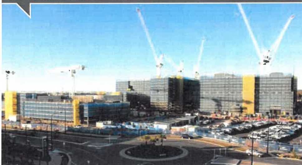
Kwikform: Sunshine Coast University Hospital; South East Queensland
