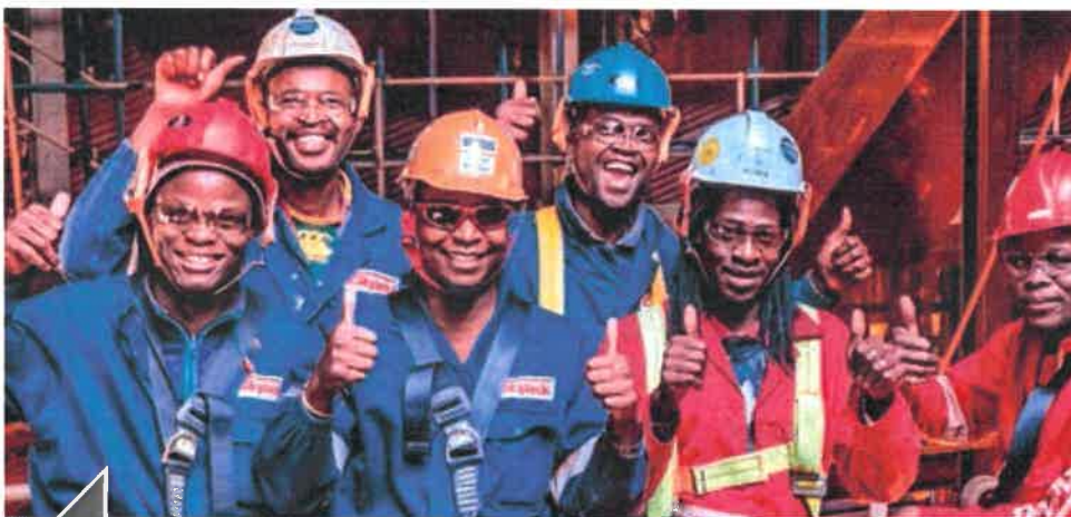
Skyjacks: Suspended access site crew working at Kusite Power Station, South Africa.
