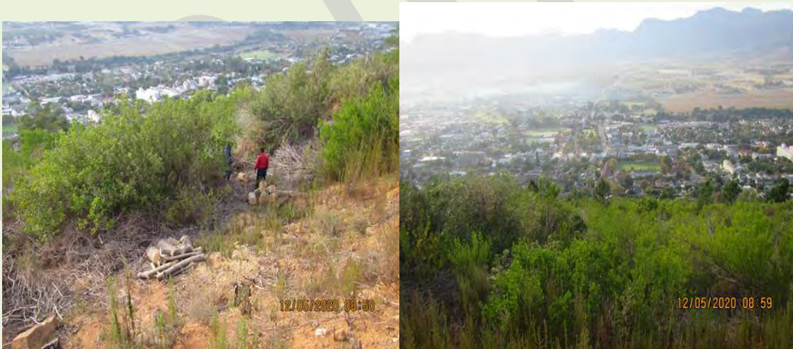
Pictures taken during clearing (above)
